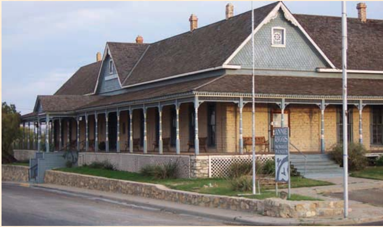
The adobe hotel with Victorian detailing was built in 1899 and has housed the Annie Riggs Memorial Museum since 1955.
